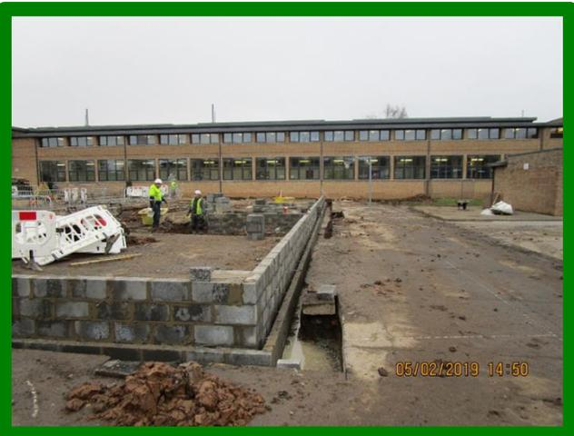
Work on the new extension continues, with substructure masonry commencing this week – this is moving on a pace, with the amount of brickwork growing every day.
